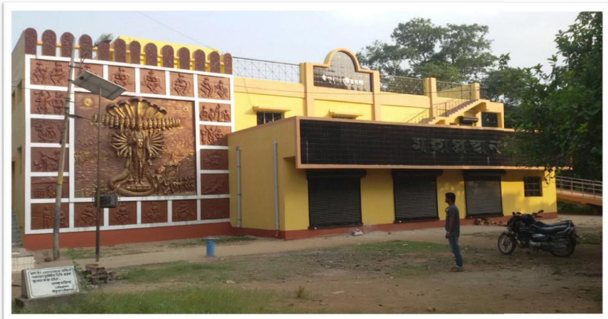
Crematorium:- Construction is in progress.
